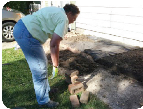
Janet Ford places brick to line the new landscaping.
